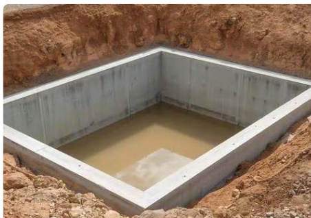
Underground water tanks
