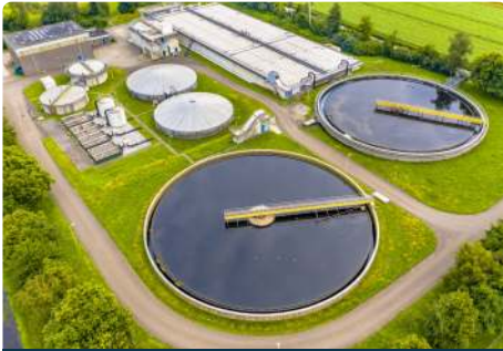
Water & waste water treatment plants
