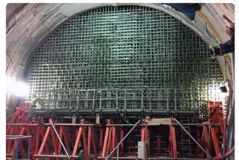
Tunneling & temporary reinforcement
